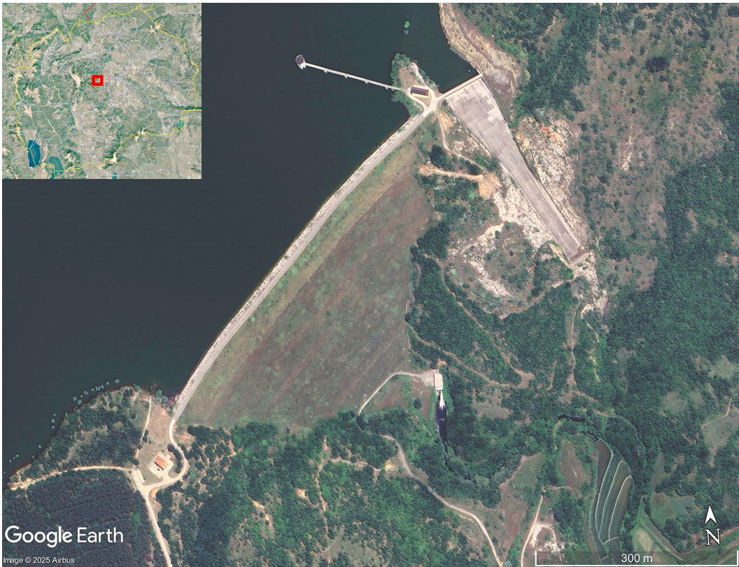
Figure 1: Satellite image of the Lisiche embankment Dam (Google Earth, 2025).
