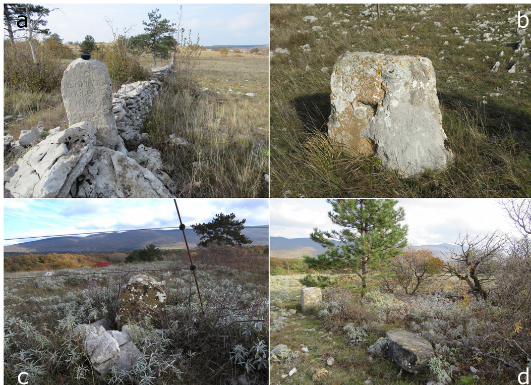
Figure 16: Different types of boundary marks on the north-eastern border of the cadastral municipality of Črnotiči: a) carved boundary mark with inscriptions in Krapnik from 1819; b) limestone boundary mark with the year 1865 below Črnotiči airport; c) above the area named Trpce: a roughly carved boundary stone without inscriptions made of sandstone (No. 7 in Figure 12); and d) Soligrad: on the left, an Italian concrete trigonometric pillar and, on the right, an uprooted boundary stone made from sandstone (photo: M. Triglav Čekada, 2023).
