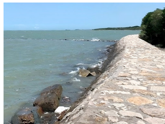
Figure 3: Stone embankment at Thanh An Island.
