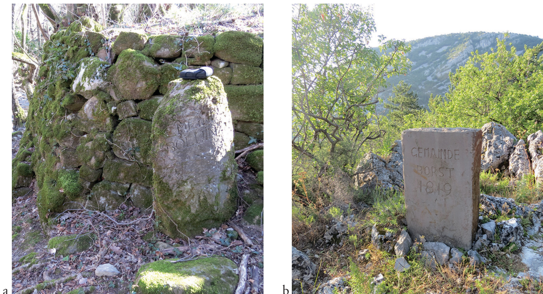
Figure 4: The cadastral municipalities boundary stones: a three-sided stone in village of Botač (Table 1, No. 9) and a two-sided stone under the Sveti Mihael hill (No. 12).
